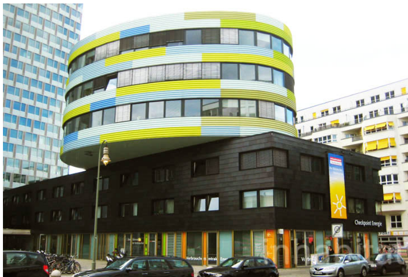
Figure 5.5: GSW Headquarters has a passive ventilation system which reduces the energy demand [47]
