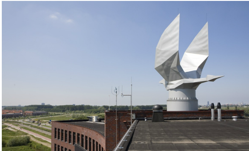
Figure 5.8: Stadsdeelcomplex Leidschenveen-Ypenburg with a wind cowl improving natural ventilation [51]
