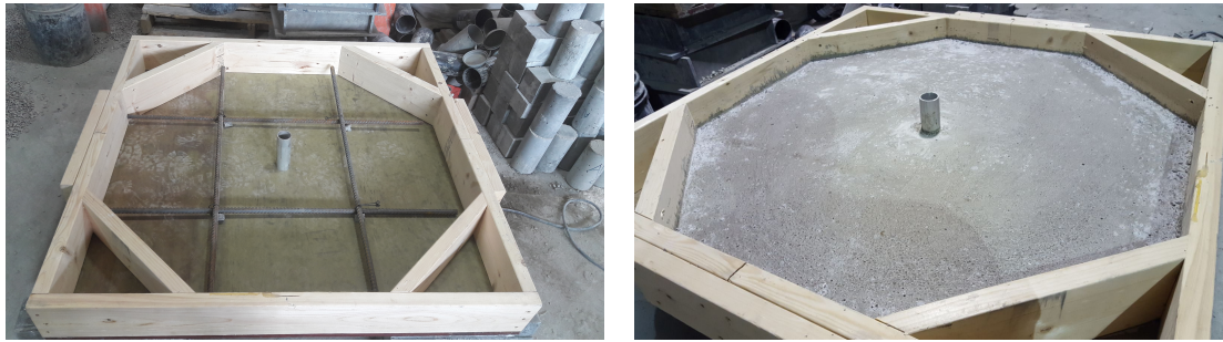
(a) Concrete pouring form work
