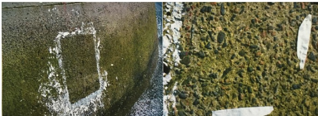
Figure 2.1: Abrasion damage to the Confederation Bridge [Newhook and McGuinn 2007]
