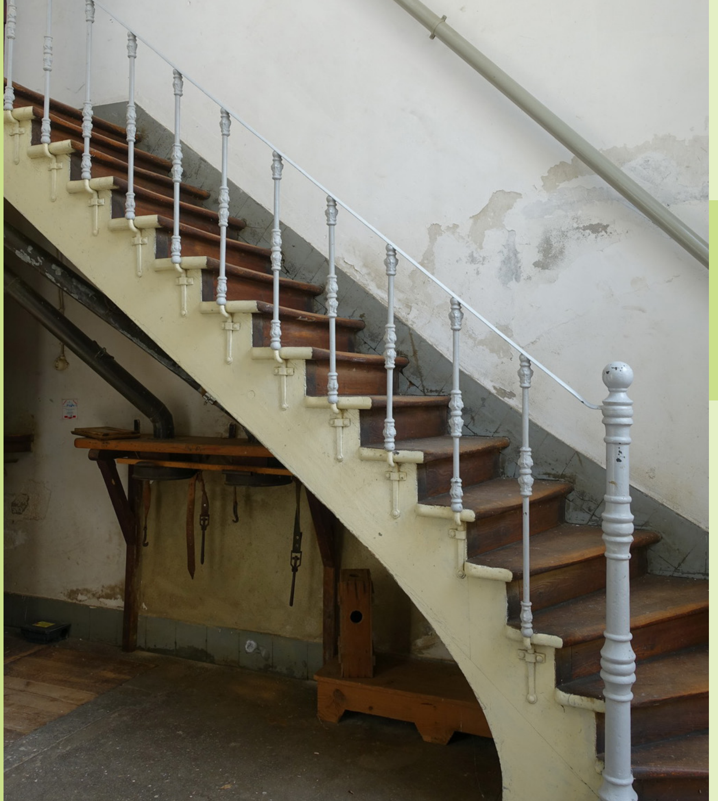
Image Staircase silos milling (photo by Hielkje Zijlstra, 04-09- 2016)
