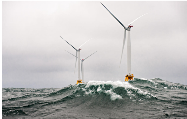
Figure 1.3: Floating horizontal axis wind turbines (HAWTs) [21]. The photograph is taken by Dennis Schroeder / NREL.
