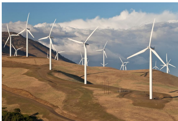
Figure 1.1: Wind farm of horizontal axis wind turbines (HAWTs) [11]. The photograph is taken by Inga Spence / Alamy Stock Photo.
