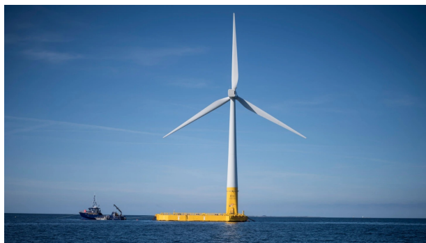
Figure 2.7: A floating, conventional horizontal axis wind turbine is placed offshore near Le Croisic, western France [38]. The photograph is taken by Sebastian Salom Gomis.
