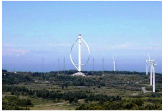
Figure 2.10: The Lavalin Éole is the largest VAWT, standing in Québec, Canada. It is a Darrieus wind turbine [43].
