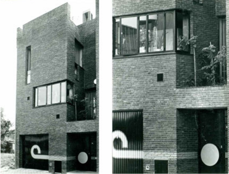
FIG. 8 Woning Gardeline, Isidoor Devosstraat, Sint-Amansberg (Gent), 1968-69, Architect BARO / Eric Balliu & Johan Baele [Foto: Archief BARO, Jul Vandeveldel]
