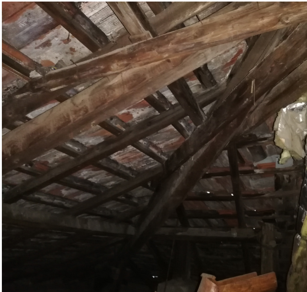
Figure (67) : Internal roof structure (Survey Document) (Personal Document)
