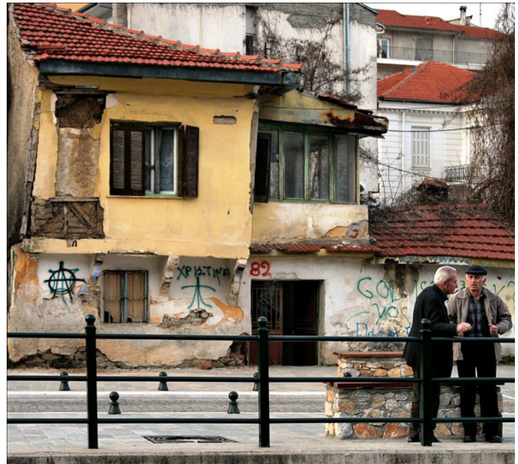
Figure (57): View from the street in the historical centre of Florina showing buildings influenced by the Turkish Occupation ( https://www.dpgr.gr/forum )
