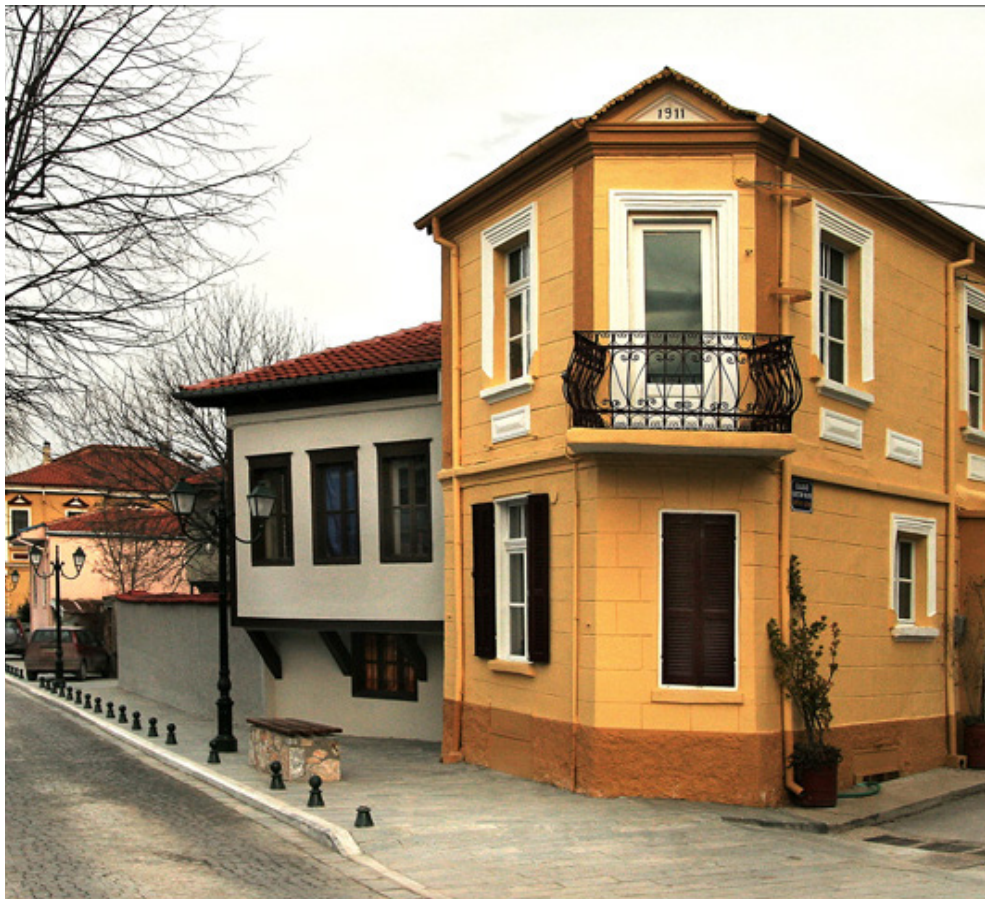
Figure (54): View from the street in the historical centre of Florina showing two types of heritage structures: the yellow is considered neoclassical and the white one is influenced by the Turkish Occupation ( https://www.dpgr.gr/forum )
