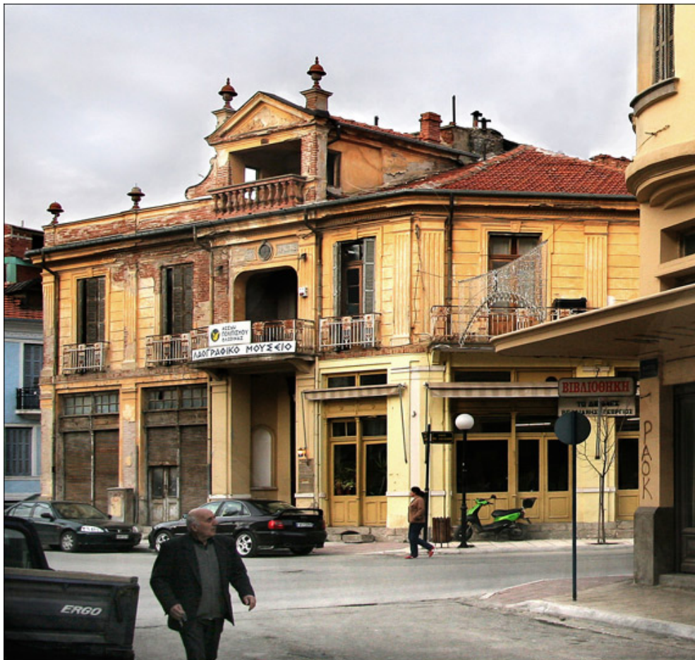
Figure (72) : Current Status of building "Diethnes" ( https://www.dpgr.gr/forum )
