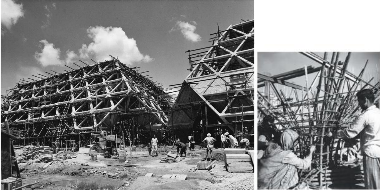
Figure 6, 7. Halls of Nations and Industries under construction (Mahatta, 2020).
