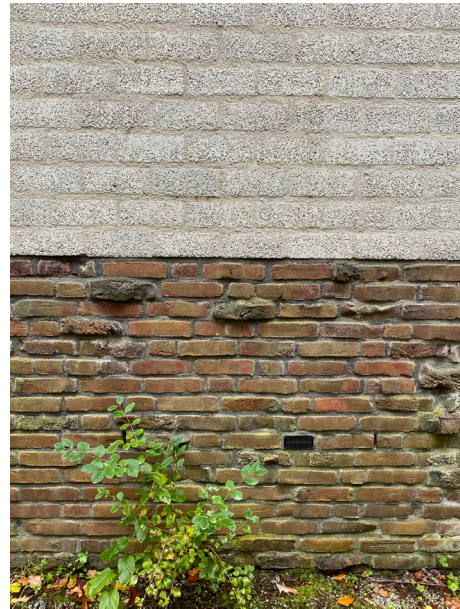
The materials of the existing institution like building: the bricks have natural shapes and are weathered
