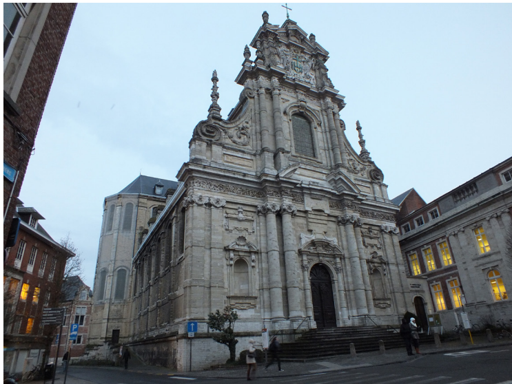
9. Top: Floor plan of Saint Michael's church in Leuven. Bottom: Entrance of Saint Michael's church in Leuven.
