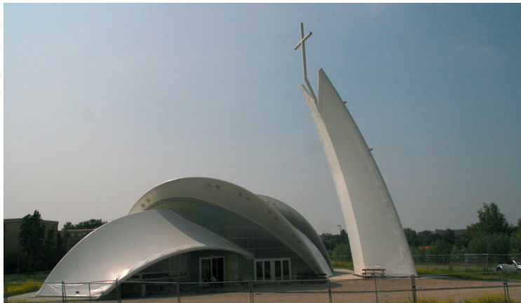
61. The steel structure covered with a white teflon material.
