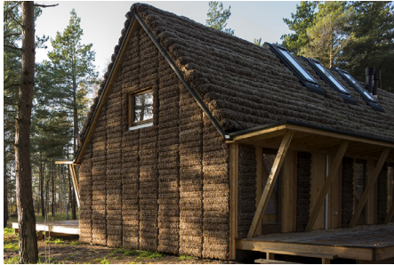
Figure .... The Modern Seaweed House. (Vandkunsten Architects, n.k.)
