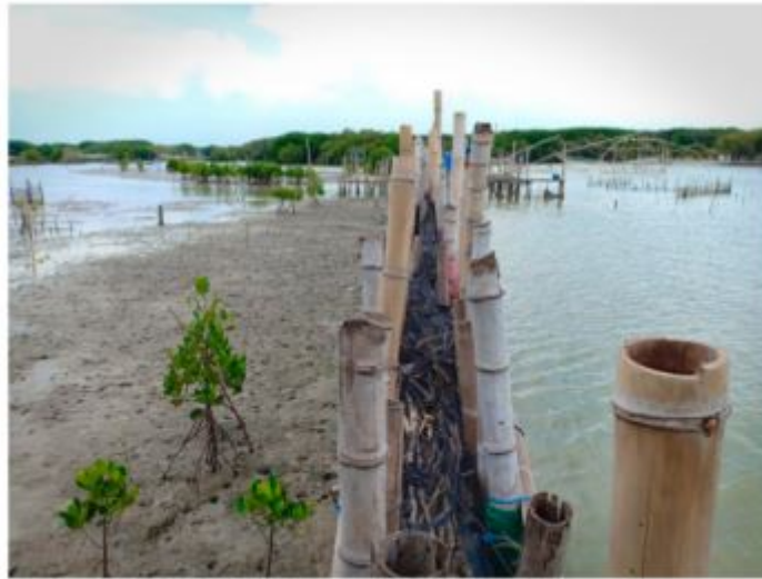
Figure 1.4: Sideview of permeable dam filled with brushwood. With on the left sheltered area and on the right is the open sea. From Winterwerp et al. (2020)
