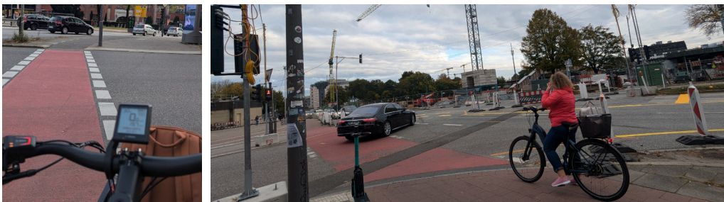
Figure 20. Multiple mobility hotspots under construction during the visit resulted in inconsistent bike lanes.
