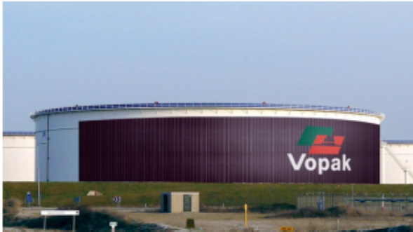
Figure 1.4: Thin-film application on Vopak terminal [10]
