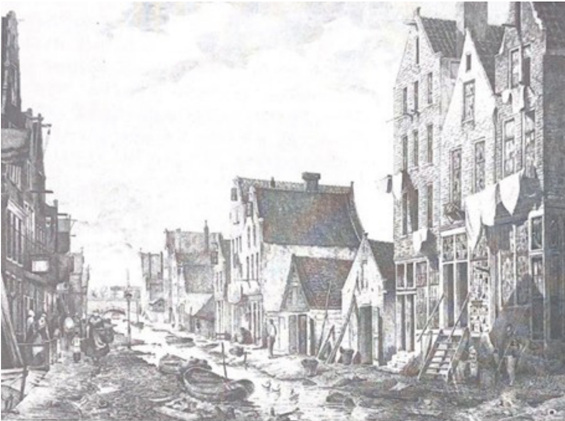
Image 3. Neglected and dilapidated working-class houses in the Jordaan (Amsterdam). (Prak, 1991)
