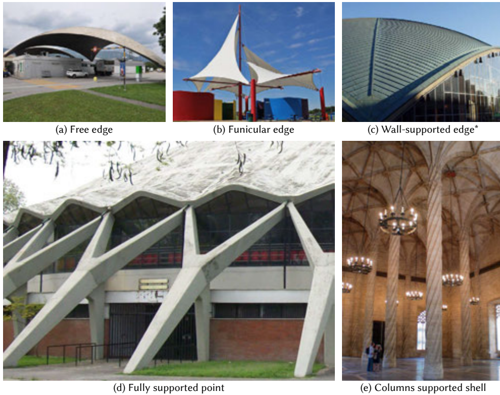
Figure 2.8: Examples of boundaries and supports. (a) Raststätte Deitingen [Deitingen Service Station], Deitingen, Switzerland. (b) Celebration Park, Allen, Texas, United States. (c) Kresge Auditorium*, Cambridge, Massachusetts, United States. (d) Palazzetto dello Sport [Small Sport Palace], Rome, Italy. (e) Llotja de la Seda [Silk Exchange], Valencia, Spain. [Source: (a) Peter Eigenraam; (b) PFEIFER FabriTec; (c) Daderot@commons.wikimedia.org, licensed under CC BY-SA 3.0; (d) Blackcat@commons.wikimedia.org, licensed under CC BY-SA 3.0; (e) TMaschler@commons.wikimedia.org, licensed under CC BY-SA 3.0]
