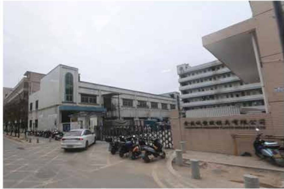
Figure 6.19 Pictures of Buildings needed to be renewed Source: map.baidu.com
