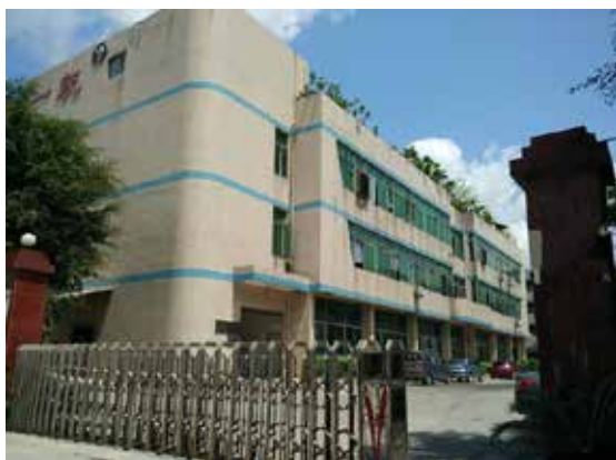
Figure 5.26 Old Industrial Park
