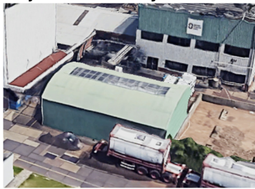
Adress: Lindtsedijk 8, Zwijndrecht Function: Oil refinery Start company: 1910 Construction year: 2022
