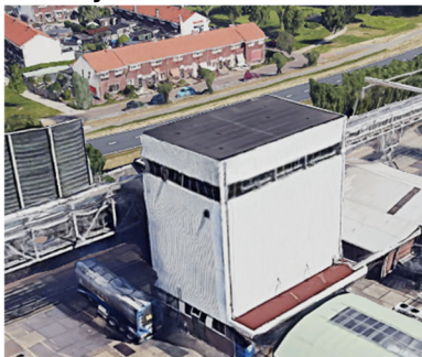
Adress: Lindtsedijk 8, Zwijndrecht Function: Oil refinery Start company: 1910 Construction year: 1978
