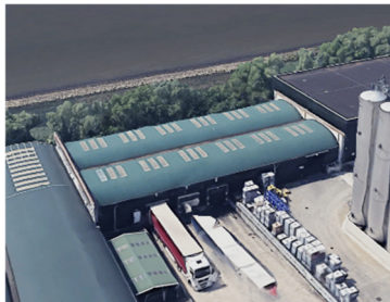
Adress: Merwedeweg 17, Zwijndrecht Function: Lubricant industry Start company: 1891 Construction year: 2000
