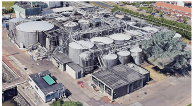
Adress: Lindtsedijk 8, Zwijndrecht Function: Oil refinery Start company: 1910 Construction year: 1960
