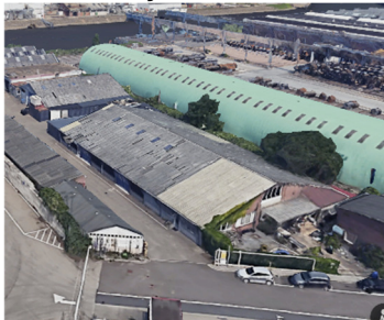
Adress: Oudemaasweg 5, Zwijndrecht Function: Ship engine supplier Start company: 1939 Construction year: 1954
