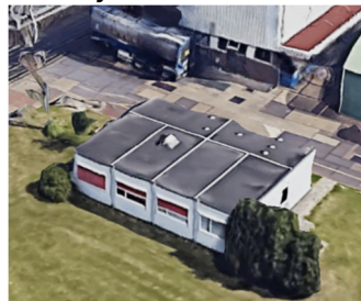
Adress: Lindtsedijk 8, Zwijndrecht Function: Oil refinery Start company: 1910 Construction year: 2004
