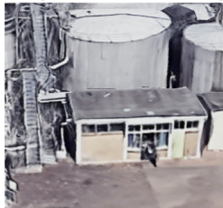
Adress: Lindtsedijk 8, Zwijndrecht Function: Oil refinery Start company: 1910 Construction year: 1960
