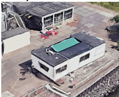
Adress: Lindtsedijk 8, Zwijndrecht Function: Oil refinery Start company: 1910 Construction year: 2022
