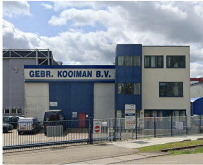
Adress: Lindtsedijk 78, Zwijndrecht Function: Shipwarf Start company: 1884 Construction year: 1980
