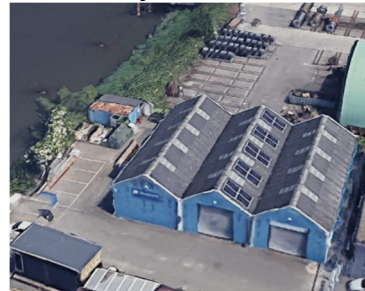
Adress: Oudemaasweg 5, Zwijndrecht Function: Ship engine supplier Start company: 1939 Construction year: 1954
