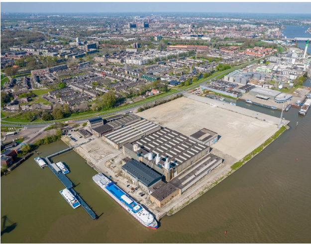
Figure 14: Drone picture of Schokbeton site (PIER14, n.d.)
