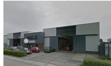
Adress: Merwedeweg 12, Zwijndrecht Function: Woodworkers Start company: 2012 Construction year: 1985
