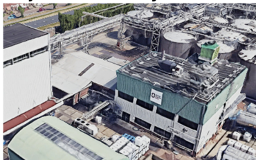
Adress: Lindtsedijk 8, Zwijndrecht Function: Oil refinery Start company: 1910 Construction year: 1978
