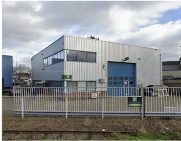
Adress: Noordweg 21, Zwijndrecht Function: Hydraulic installations Start company: - Construction year: 1994
