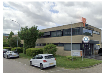
Adress: Merwedeweg 5, Zwijndrecht Function: Industry Start company: 1957 Construction year: 1969
