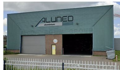
Adress: Merwedeweg 9, Zwijndrecht Function: Aluminium production Start company: 1987 Construction year: 1980
