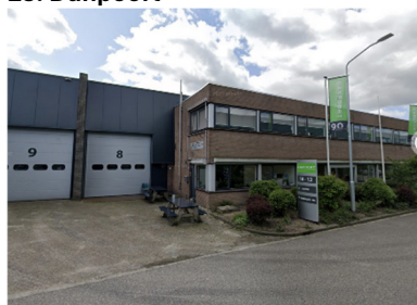
Adress: Kilweg 6, Zwijndrecht Function: Abrasives producent Start company: 1932 Construction year: 1980
