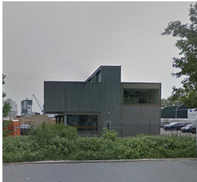
Adress: Merwedeweg 20, Zwijndrecht Function: Wood supplier office Start company: 1949 Construction year: 2011
