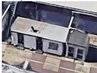
Adress: Lindtsedijk 8, Zwijndrecht Function: Oil refinery Start company: 1910 Construction year: 1960
