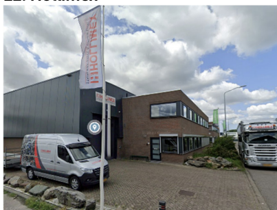
Adress: Kilweg 2, Zwijndrecht Function: Steelproduction Start company: 1980 Construction year: 1980
