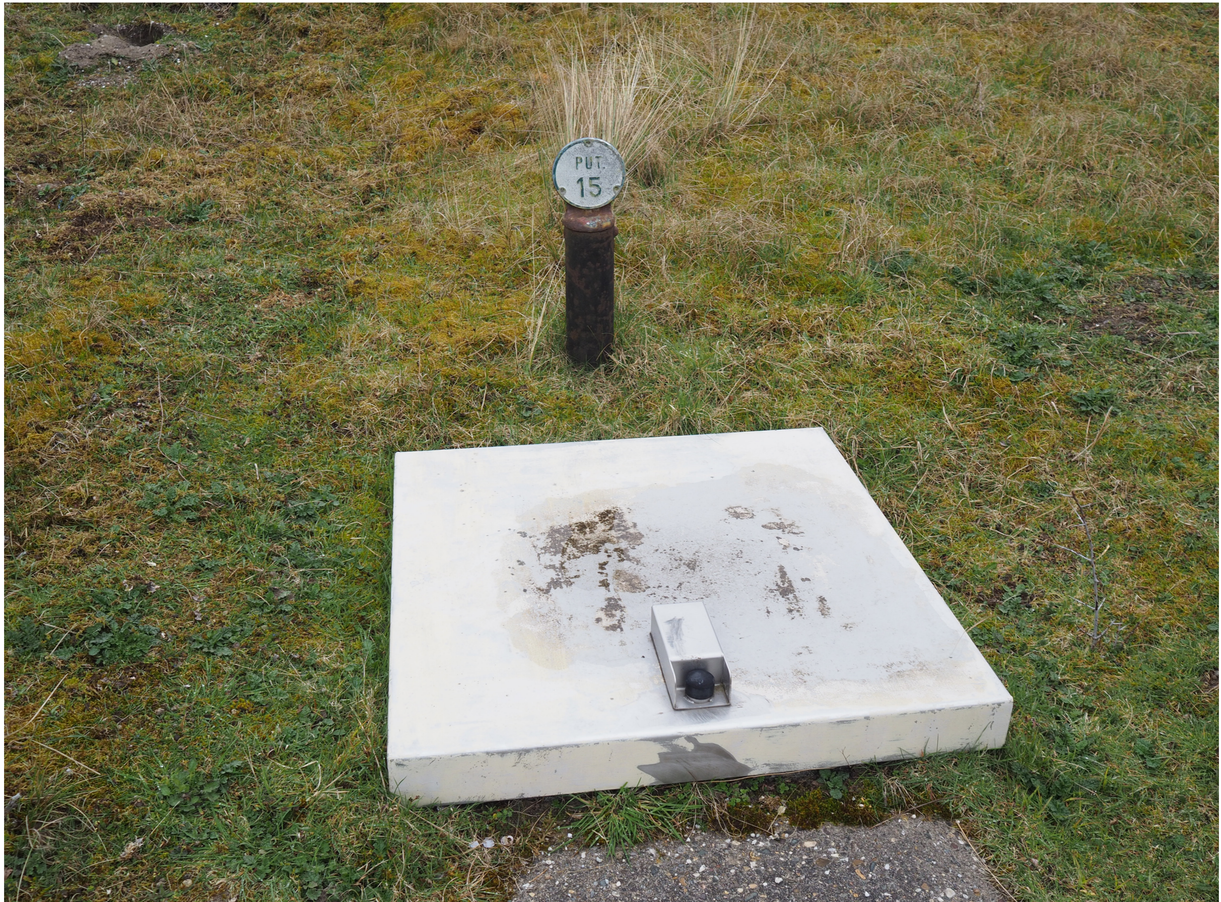
Water Well Water well of the company
