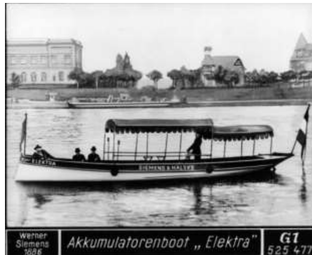
Figure 73: Elektra (1886) was the first battery powered vessel [Ref: siemens.com].
