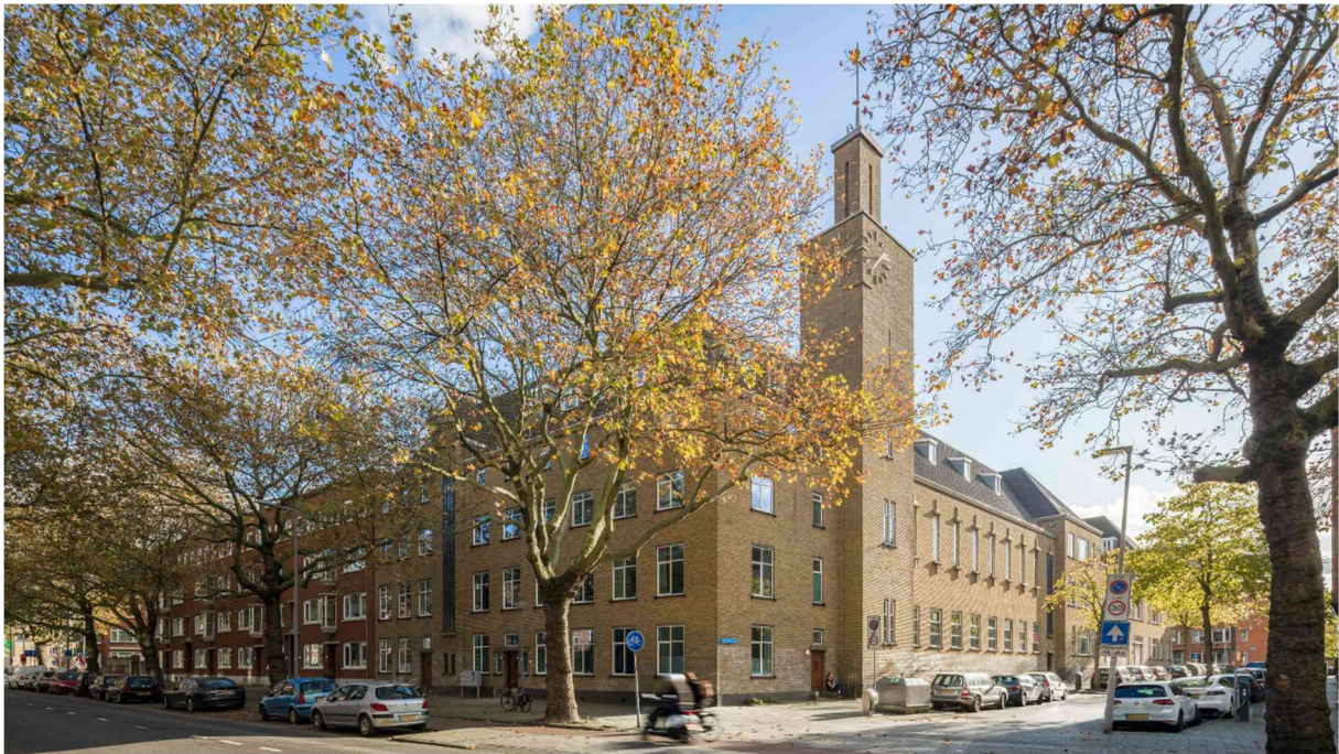
Figure 21. Rotterdamse School, prior to construction of the front doors in the chapel. (EGM architecten, n.d.).
