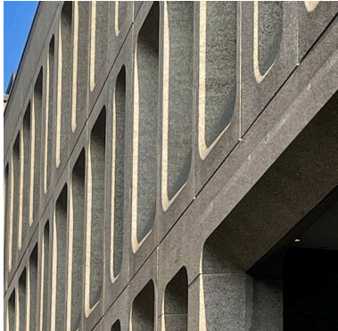
Daylight of facade niches
