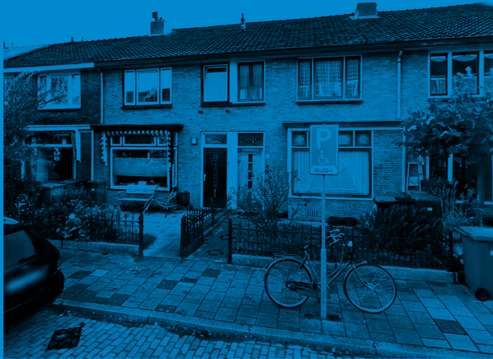
01. Context: the window will be repaired in situ. Demolition is prevented
