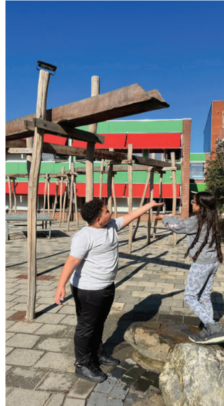
By disconnecting drainpipes, the rainwater is led directly to the playground through these wooden construction
