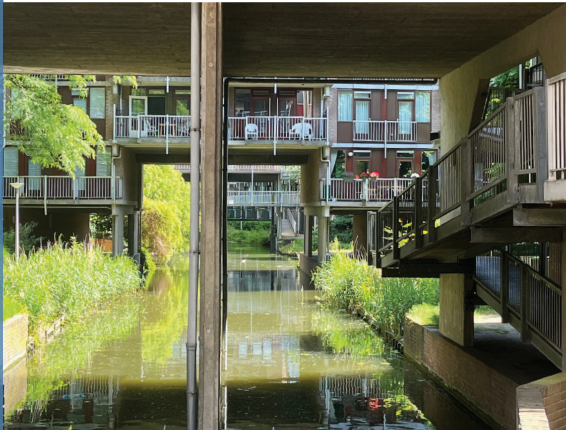
Rainwater is filtered by the reed bed system
