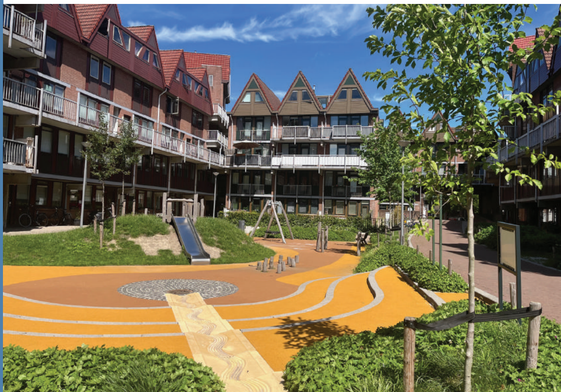
Rainwater from disconnected drainpipes flows to the well via 'stairs'
