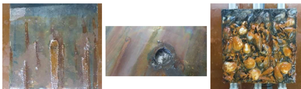
Figure 13. Marine growth covered plate after three weeks of accelerated corrosion.
