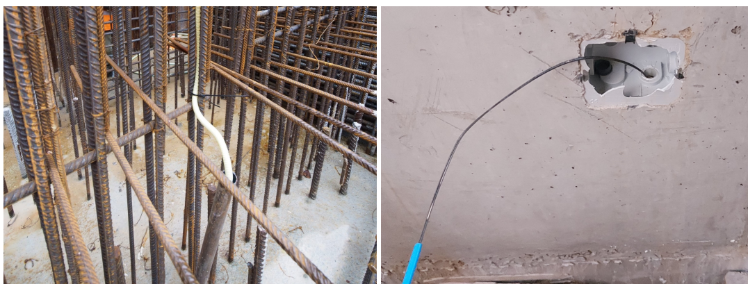
(a) FO access on the surface.
