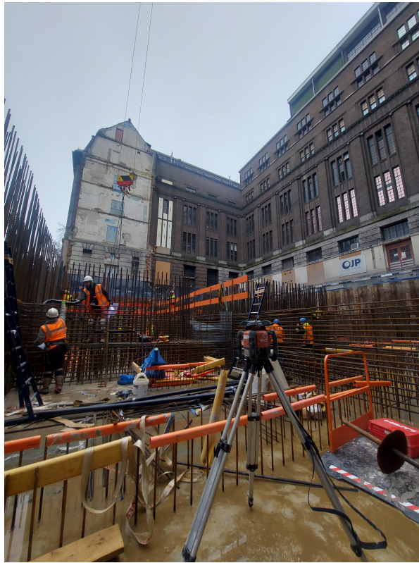
Figure B.6: Basement slab is visible.
