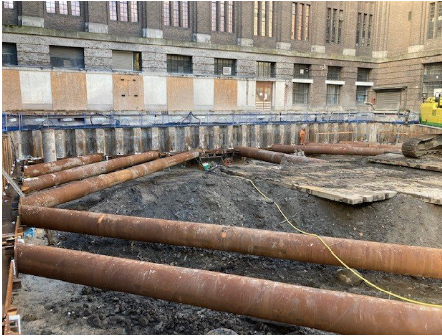
Figure B.4: Installation of struts at -2.0 m (from The POST Bouw, 2023).
