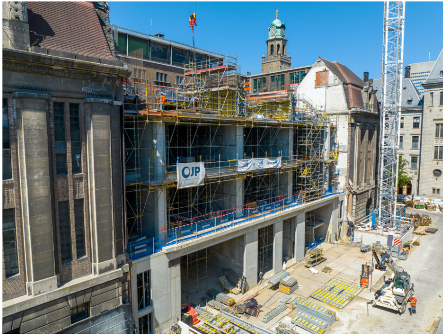
Figure B.8: Groundfloor and first two floors are built (from Arch Daily, 2023).
