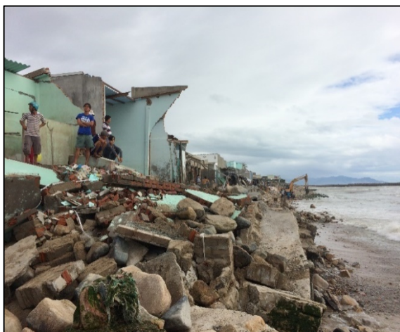
a. Houses are damaged by erosion.
