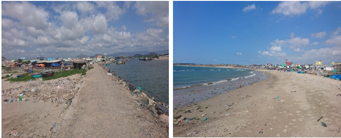
c. A dike near the estuary
