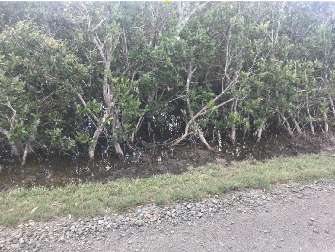
Figure 1: 21 st March 2019 Super full moon spring tide (3.8m above MLLW). Access road erosion also observed. This has accelerated (see next figure)
