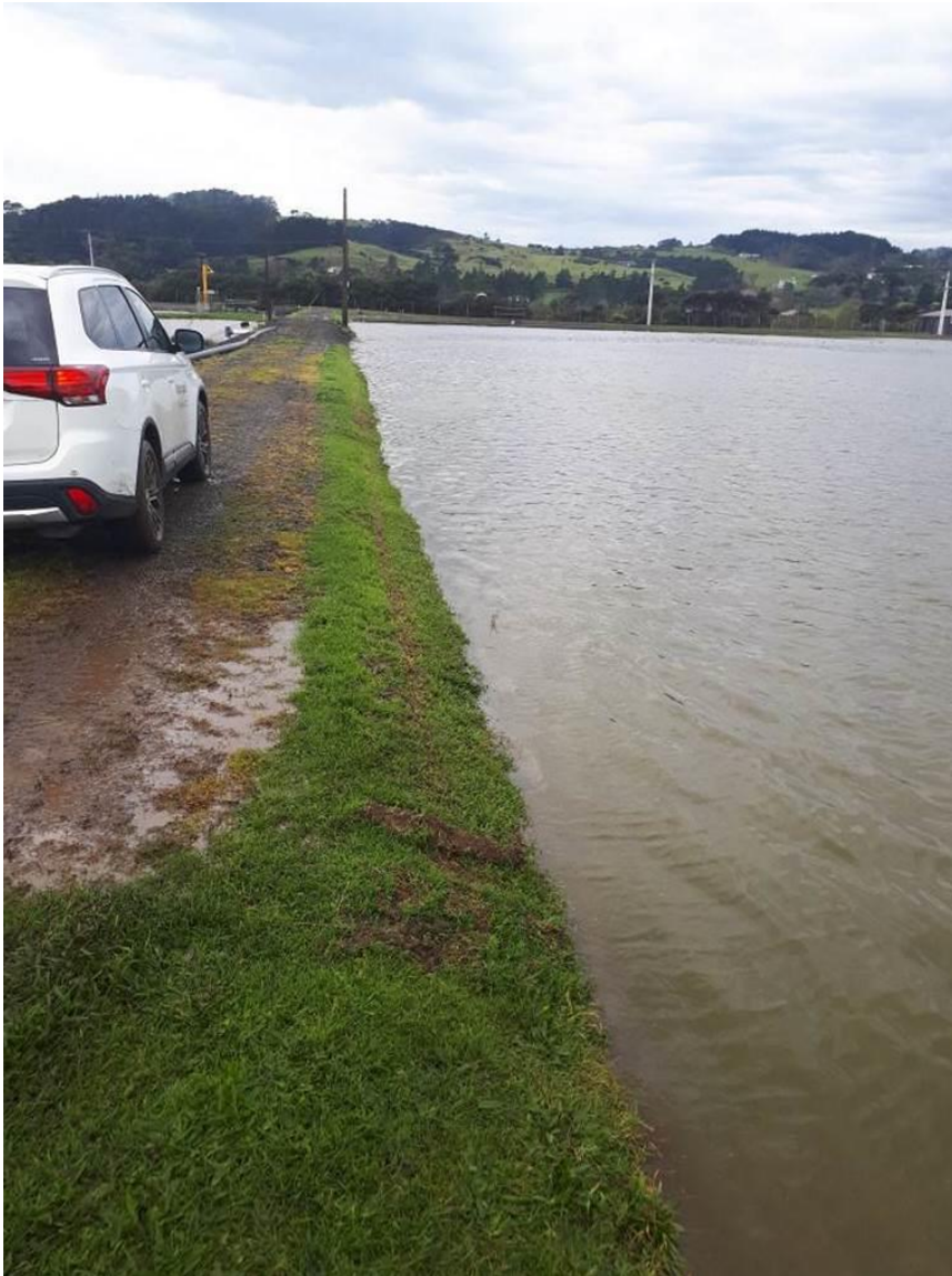
Figure 2: 9 th September 2017 wet weather event (125mm between 3 rd and 11 th Sep). Pond levels at 1660mm. The pond will overtop the dam embankment into the harbour at 1.85m.
