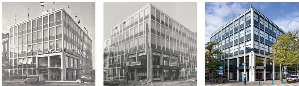
Figure 3: left photo – newspaper office “De Rotterdammer” & “Trouw” (original design, 1958), middle photo - newspaper office “Het Vrije Volk” (1979), Police office (1993 – now).
