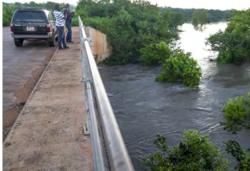
(a) Inundating floodplains at the Dome discharge station (1/2) (own work)
