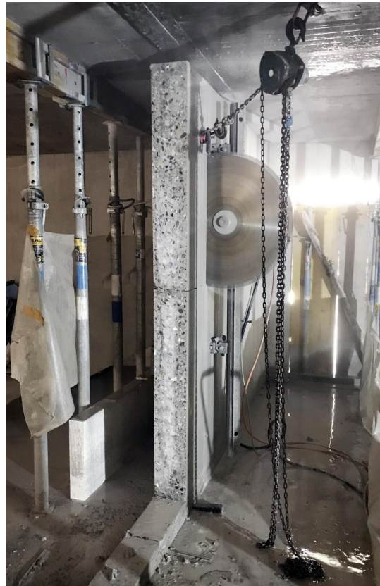
Figure 2.5: Sawing of the blocks for the Re:Crete bridge[41]
