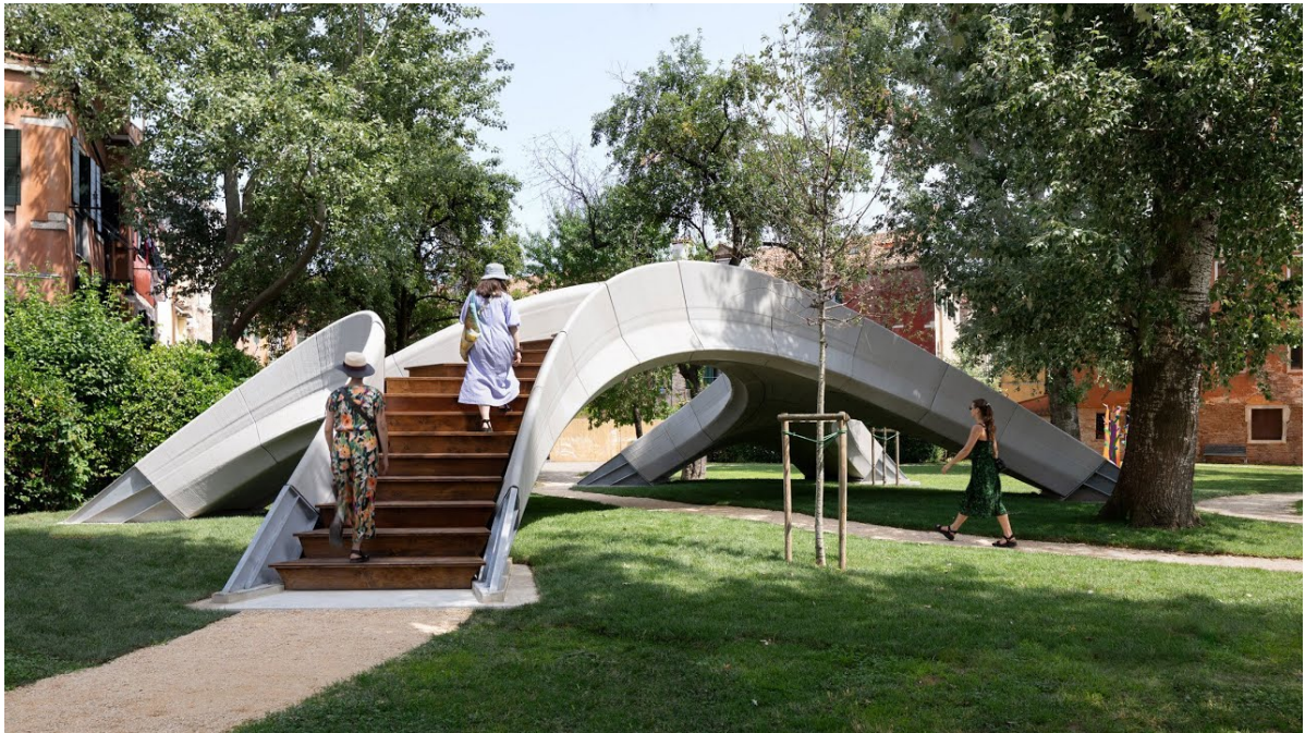
Figure 2.3: Striatus bridge made of unreinforced 3D printed masonry [40]
