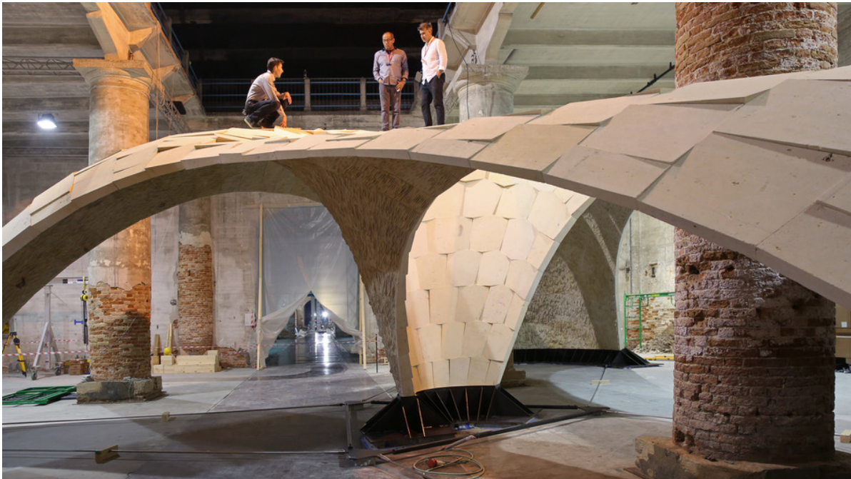
Figure 2.2: Armadillo Vault - a free-form vault made of discrete elements with no adhesives or mechanical joints [37]
