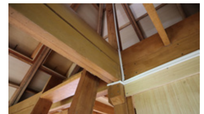
Figure 29 - Glued and screwed beams together
