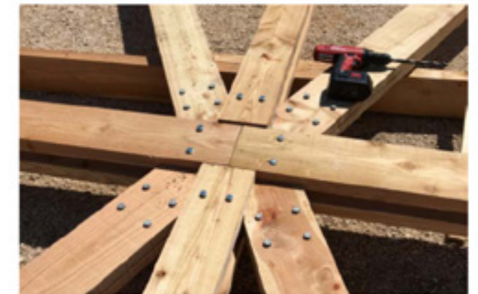
Steel-to-wood designed connections
