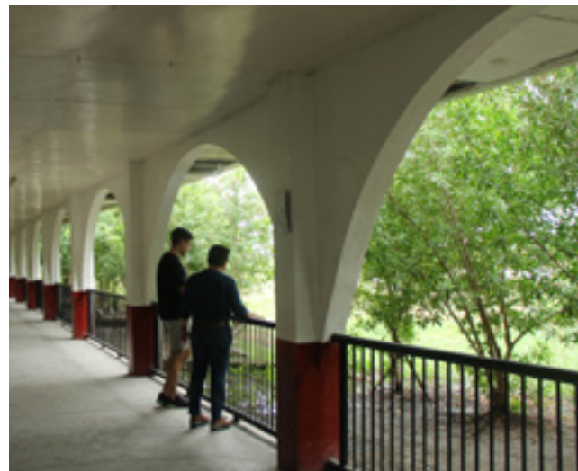
Figure 3 - Hallway behind the school
