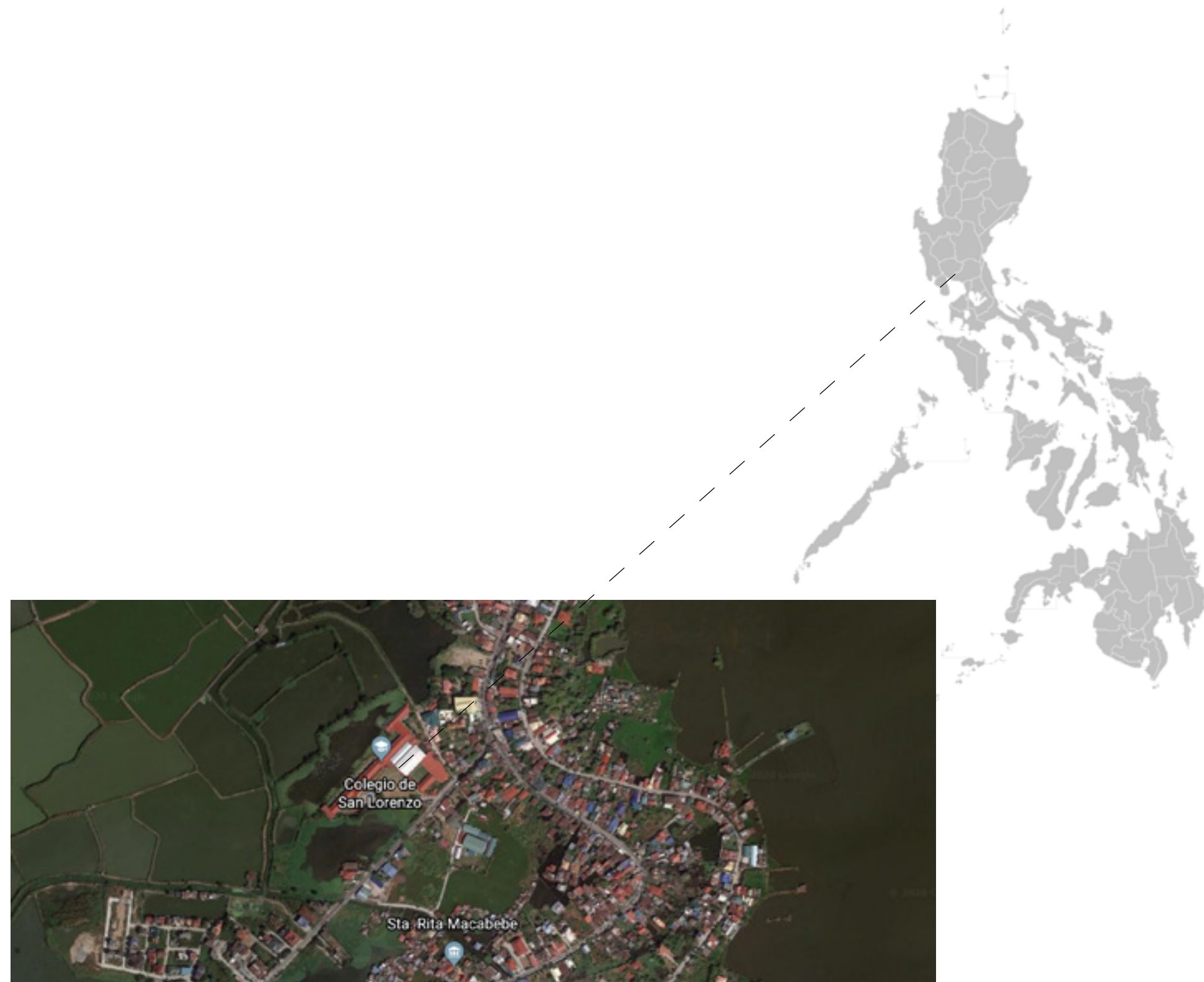
Figure 3 - Satellite view of the location of the San Lorenzo school (source: Google Earth)
