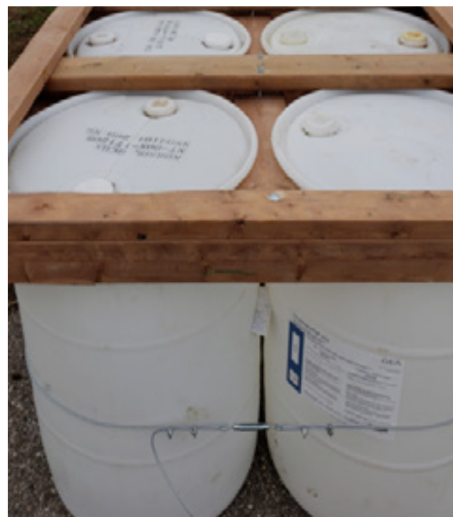
Figure 15 - Barrels secured in the frame of the NRC Pavillion (Buoyantfoundation official site)
