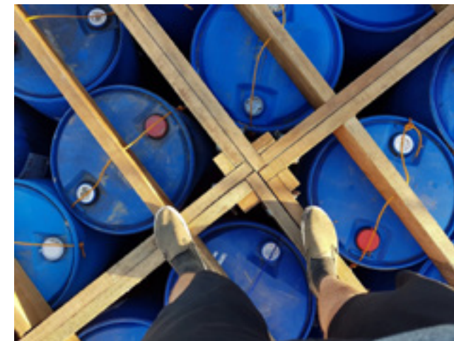
Figure 11 - Connection of barrels and double truss beams (photo by P.Ham)
