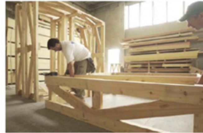
Prefabrication process off-site
