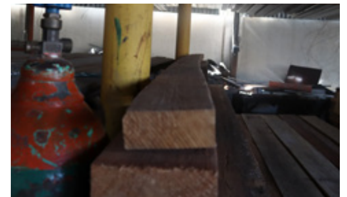
Figure 3 - Skew in the beams
