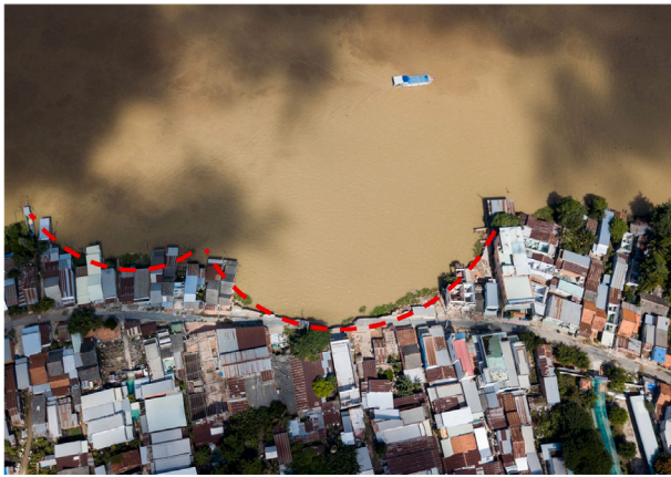
Fig. 3. Bank collapses at Mekong River, Vietnam, due to uncontrolled sand mining resulting in breaching (National Geographic, 2018, photo: Sim Chi Yin). Breaching scars are indicated with red dashed lines.
