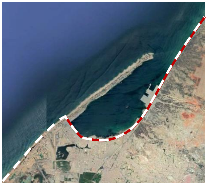
Figure 6-2 – Initial coastline used for modelling cases ShorelineS (White dashed line). White/red dashed line indicates revetment
