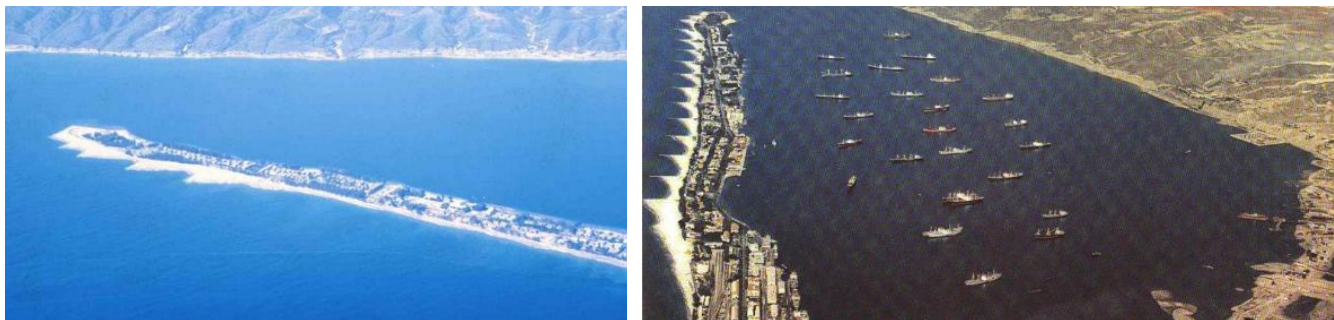
Figure 3-9 – Coastline development after construction of first 5 groynes (left) Sawtooth coastline after construction of 16 groynes. (Deltares, 2015)
