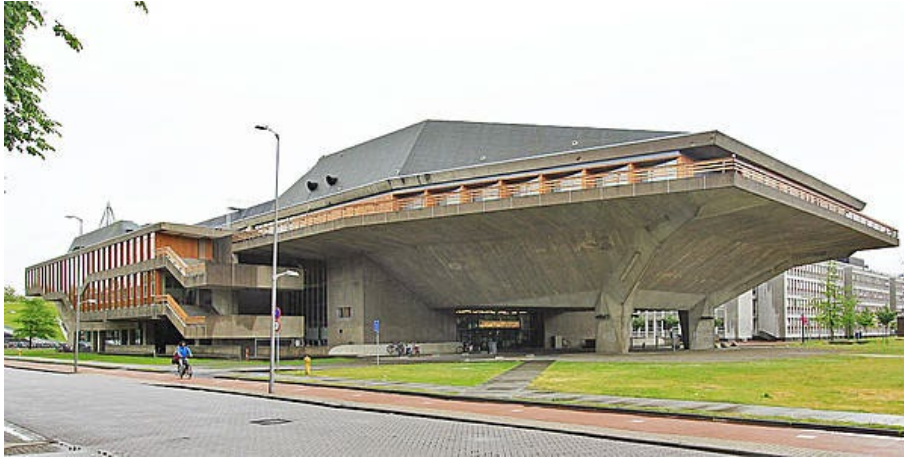
Figure 8: Picture of the front and side of The Aula showing the overhang of the auditorium (CCgrid, 2013).
