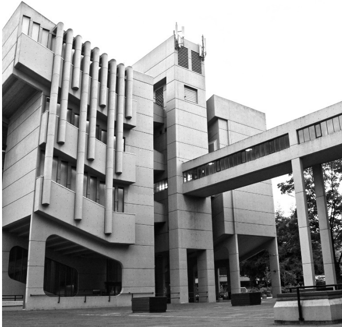
Figure 11: The Roger Stevens Building, on the right are the stacked lecture halls with the airpipes (the Culture Map, n.d.).
