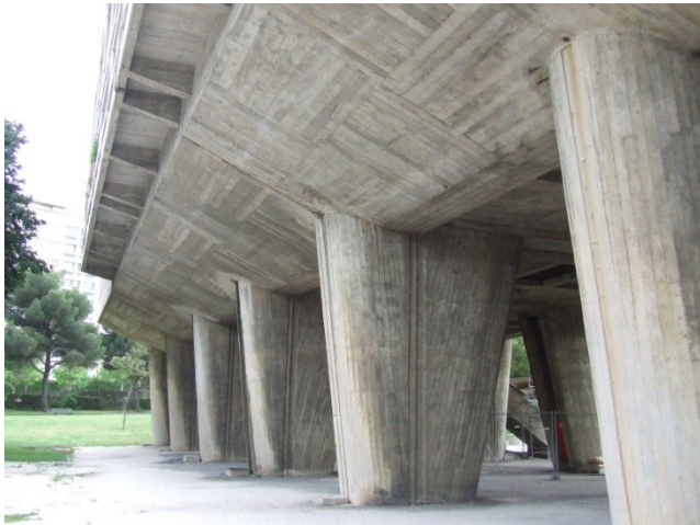
Figure 1: Béton Brut in the design of Unite d'Habitation by Le Corbusier (Glasgowfoodie, 2008).
