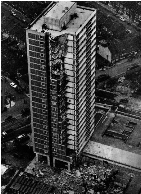
Figure 2: The partial collapse of Ronan Point (Daily Telegrapgh, n.d.)
