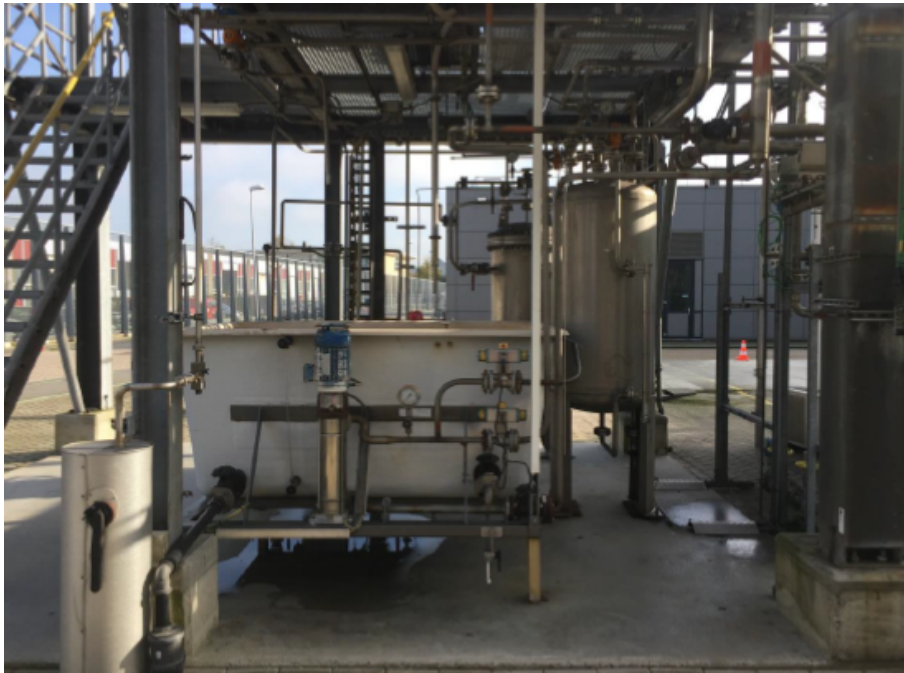
Figure 4.3: Photo of the water vessel, where the surfactant is added and mixed with the water
