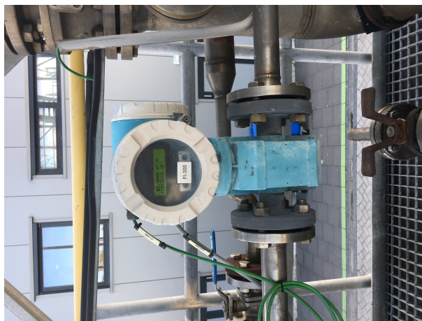
Figure 4.9: Volumetric flow meter of the water inflow
