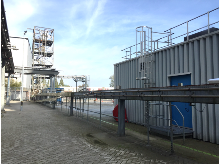
Figure 4.1: Photo of the Severe Slugging Loop at STCA
