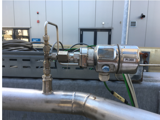
Figure 4.5: Pressure sensor PI-300 at the start of the flowline
