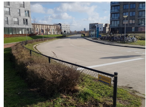
Fig. 3: Segregated bus infrastructure Almere
