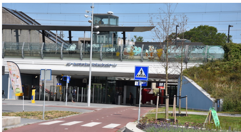
Figure 14: The western entrance of Station Holendrecht, which also visualizes the segregated traffic system. The metro and train rails above and bike and pedestrian paths underneath. From Vrijetijd Amsterdam, (n.d.).
