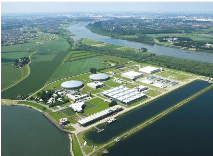
Figure 1.6. Water treatment plant in the Netherlands.
