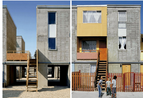
Quinta Monray buildings, incomplete houses can be filled in by the residents (2)
