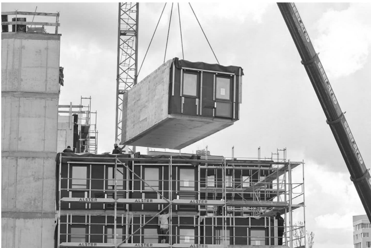
Figure 4. Modular architecture - assembling the modular unit (Jocher et al., 2018)
