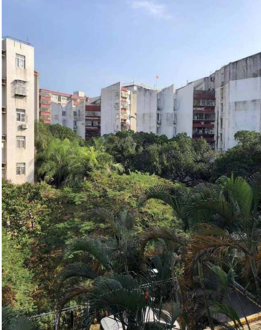
FIG. APP.B.1 Commercial housing in Nanshan district. Source: Taken by Chi Jin
