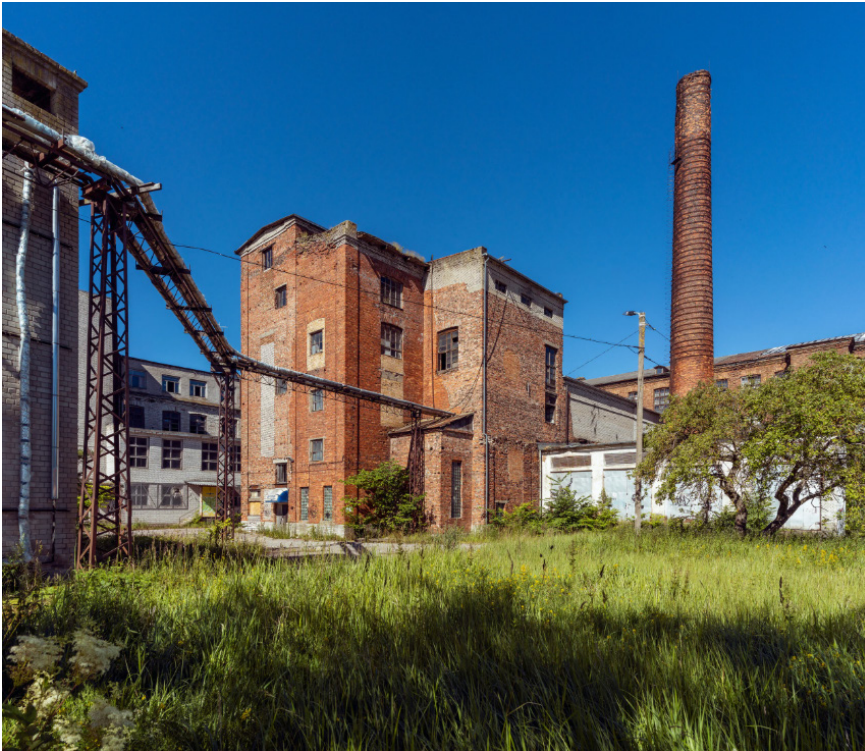
Figure 1 Current state (2023) of former boilerroom of Manufactory Quarter (KTA, n.d.)
