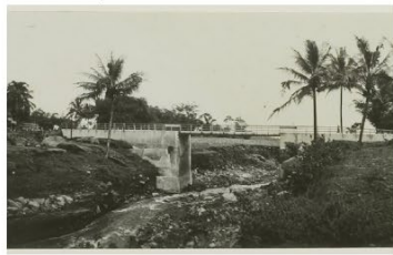
Bridge over the kali Blongkeng, Central Java - 1930
