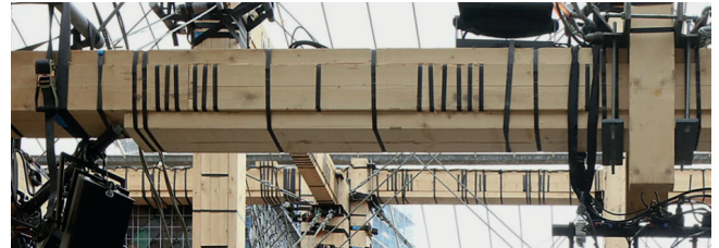
Figure 2.18: circular discrete system for peoples Pavilion in Eindhoven, using tension straps (Arup, 2017)
