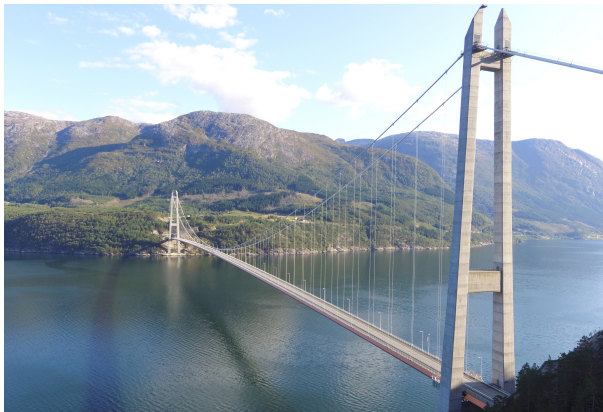
Figure 2: The Hardanger bridge (photo: Ø.W. Petersen/NTNU)
