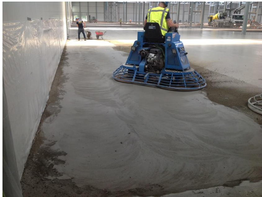
Figure 2.6 Equipment used for the monolithic finishing of the concrete surface.
