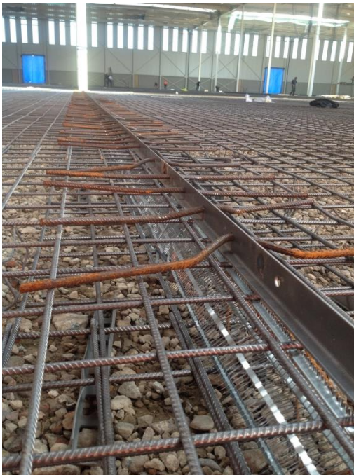
Figure 2.5 Formed joint for a hybrid reinforced concrete floor.
