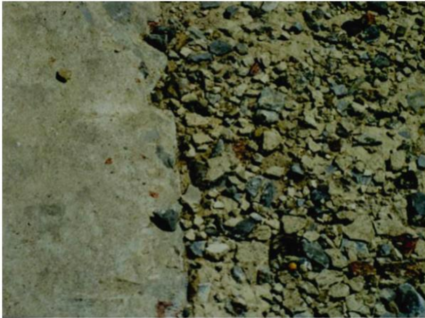
Figure 4.4 Comparison between cast-in-situ alkali-activated slag concrete (left side) and ordinary Portland cement concrete roads (right) in Ternopol, Ukraine (Provis & Van Deventer, 2014, p. 316).
