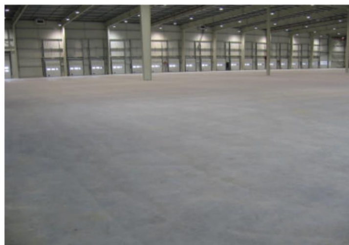
Figure 1.3 A jointless concrete ground floor (ABT, 2015c).
