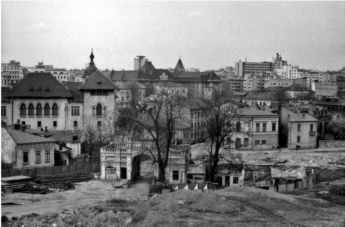
Figure 22 – Army's Arsenal partially demolished, photo taken from inside the Arsenal towards the gate and the city (Andrei Birsan, 1984)
