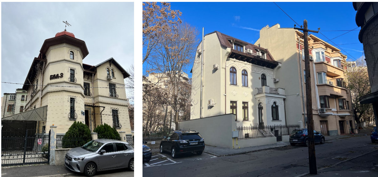
Figure 24 - Well maintained building from the neighborhood (taken by the author)
