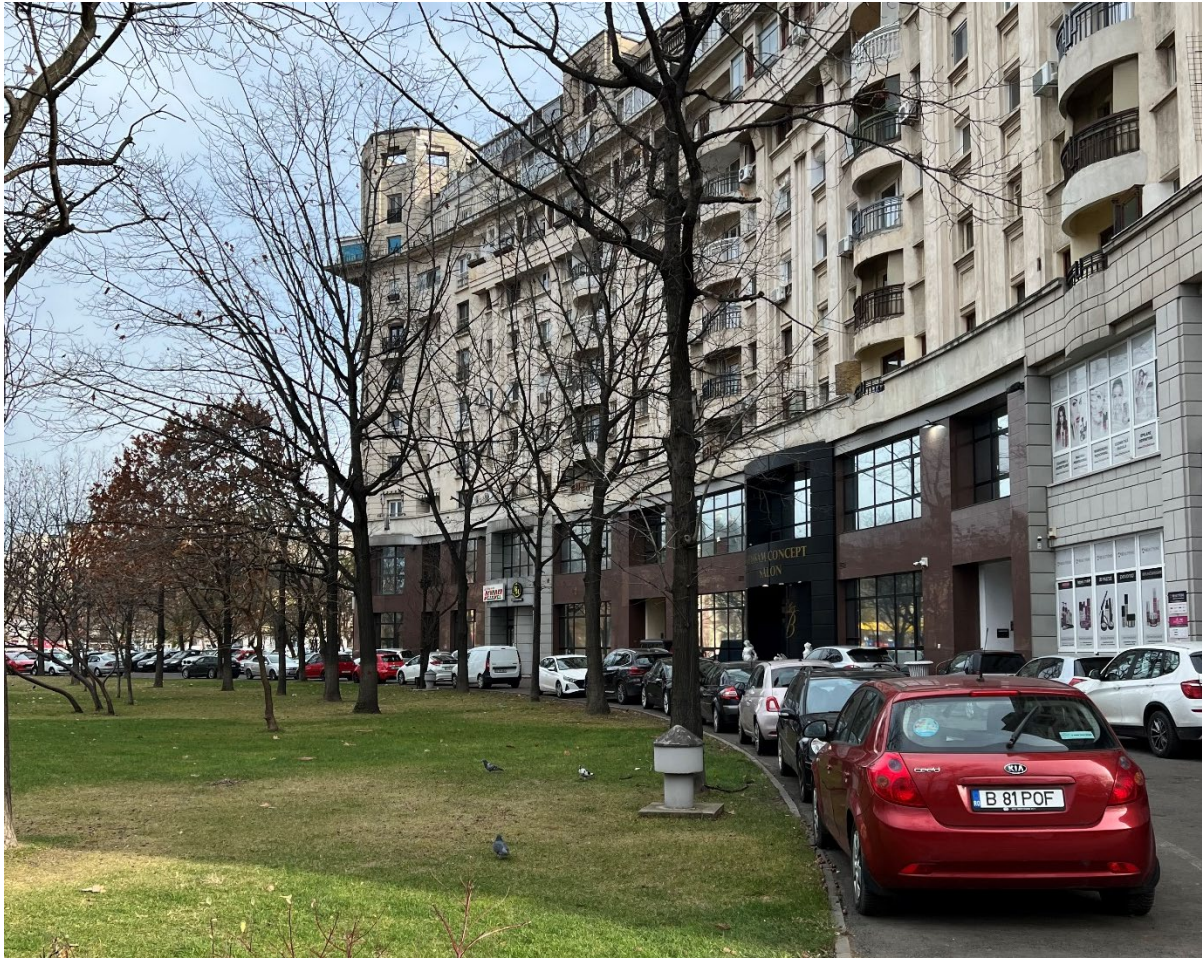
Figure 16 – Current state of the placet where Stoica used to live (taken by the author, 2023)
