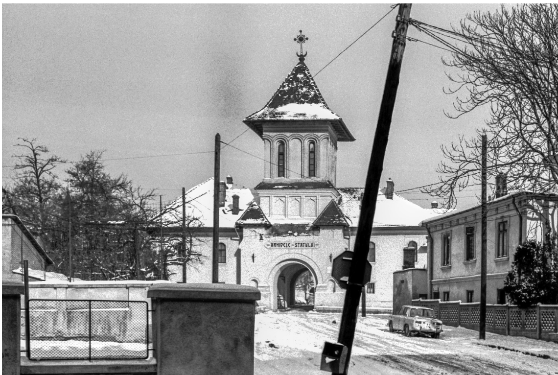
Figure 4 - Monastery Mihai Voda before demolition (Cristian Zaharia, 1978)
