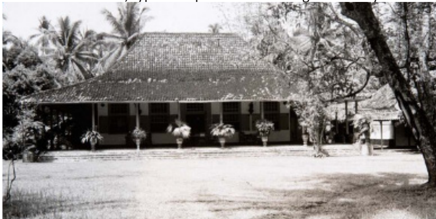
Figure 17. 'Japan' house main entrance and surroundings Indonesian colonial architecture
