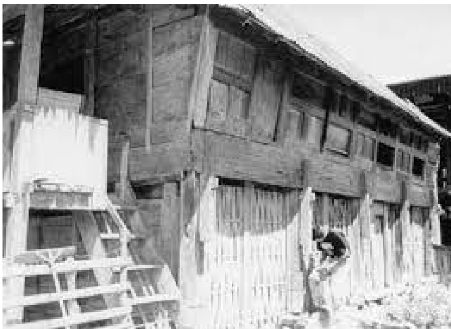
Figure 7. Sopo house using flying-planks structure
