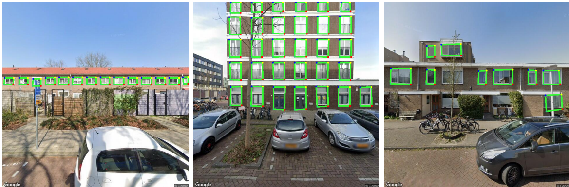
Figure 3.6: Output of the facade labeling algorithm by Li et al. [30] on street view imagery collected throughout Amsterdam.
