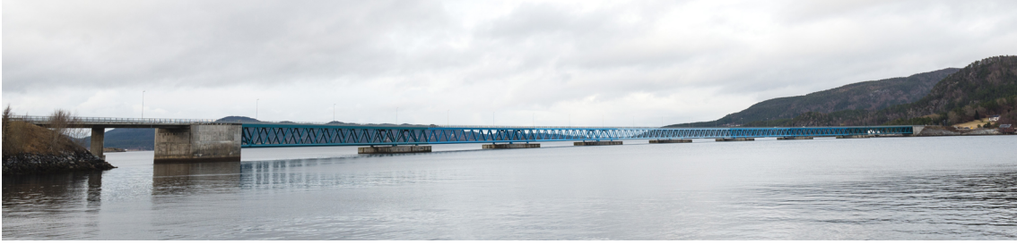
Figure 2: The Bergsøysund bridge, as seen from the south.
